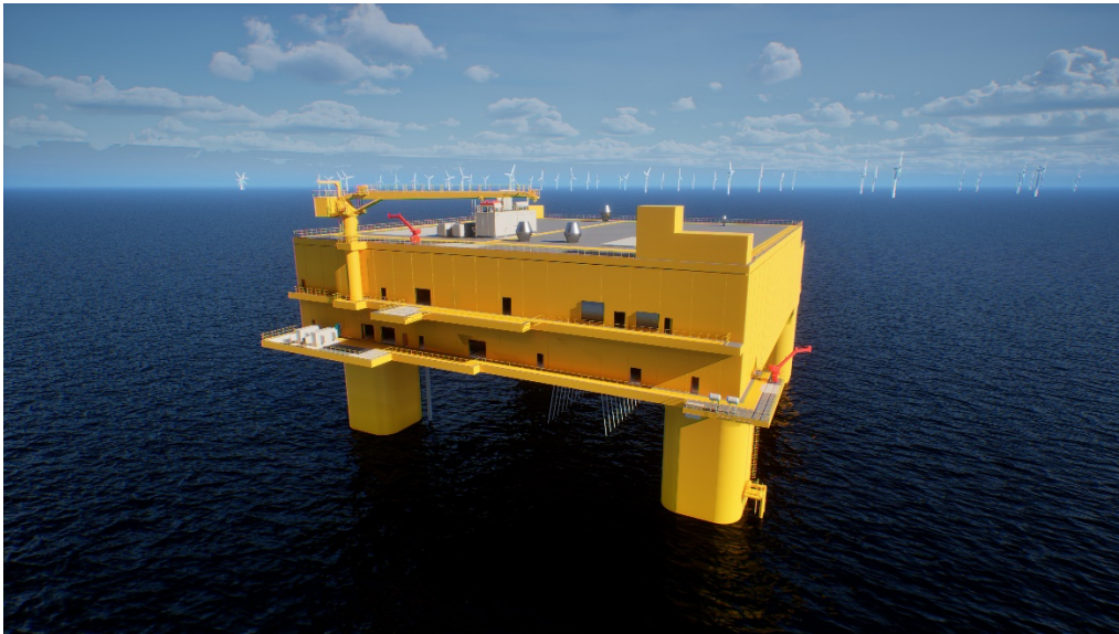
Figure 2: Zoomed-In view of floating platform with HVDC converter. Courtesy of Aibel AS and Hitachi Energy
